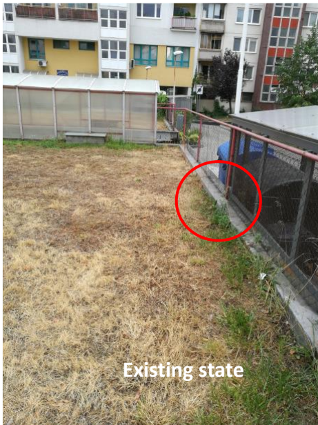
Figure 6.6.7 - Handrail incorrectly anchored to the construction; the section through the roof layers under the greenery corresponds with the existing state
