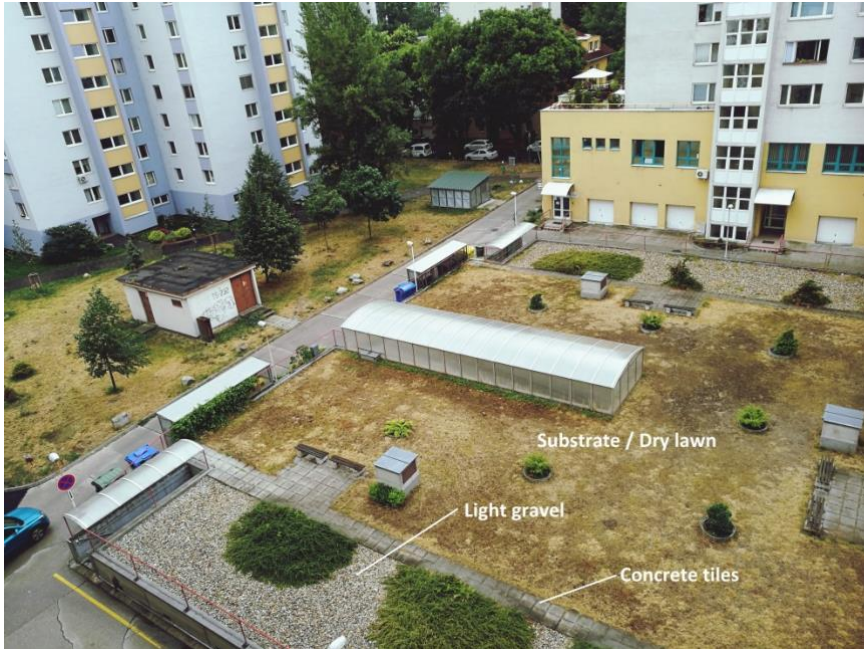
Figure 6.6.4 - Top view of the green garage roof
