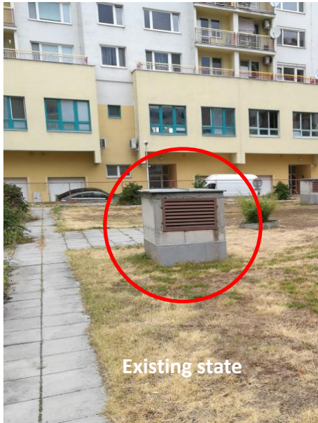
Figure 6.6.6 - Missing strip of gravel layer around the ventilation shaft; the section through the roof layers under the greenery corresponds with the existing state
