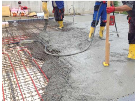
Figure 3.1.12. Laying of concrete on the pipe system and core sensors [2]
