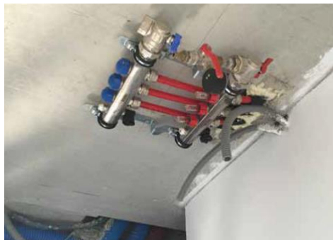
Figure 3.1.13. Installation of collector and distribution fittings [2]
