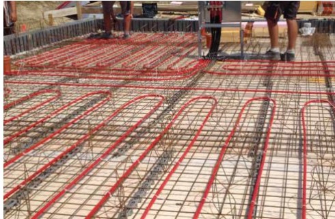
Figure 3.1.10. Laying of the pipe system [2]
