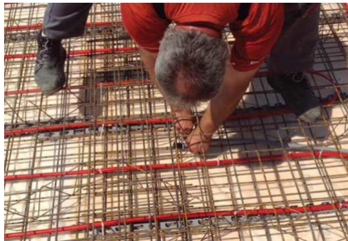
Figure 3.1.11. Installation of the core temperature sensors [2]
